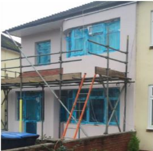
Figure 1 - External wall insulation on semi-detached dwelling
